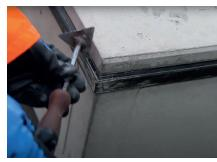
After concreting & deforming of the tunnel segment the flawless fit of the gasket has to be checked. In case that concrete slam has penetrated to the gaskets sides and surface it should be removed.
