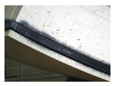
During the final control each gasket corner position should be double checked. The gasket corner should be in line with the segment corner. As well the correct type of gasket and positioning of the complete gasket in the groove should be checked. After 72 hours the adhesive will achieve it final strength, after this time the adhesive bonding should be checked visually.
