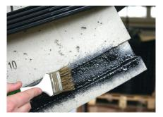
The adhesive has to be applied with a brush. It has to be applied into the groove and onto the gasket areas which have contact to the groove, especially the flanks of the gasket and groove. The adhesive should be applied equally into the groove and onto the gasket.
