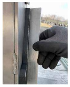
Check that the cutting surfaces are straight and even. Reconnect the assembly aid if you roughened the profile ends without assembly aid and make sure that profiles are not able to move in the assembly aid.
