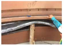
To determine the final cutting position, the start seal is fully inserted into the metal construction holding rail.
