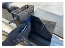
Marking the cutting positions (on both sides) with an additional length of minimum 3 cm (of combined length). Remove the gasket for cutting from the assembly aid. Cut both sides of the profile as straight as possible.
