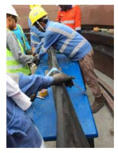
Take out the gasket from the holding metal construction rail 5 m before and after the 12 o'clock position to have enough clearance for cutting and the gluing procedure. Fix the seal at the same height as in the holding metal construction rail for better handling.
