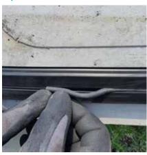
Press the remaining piece into the groove and the assembly of the round cord is finished. There must be no gap (hollow space) between the beginning and the end of the cord.
