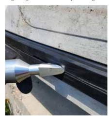
To do this, guide the line so far into the profile until you have reached the starting piece. Then take the tool out of the groove and cut the round cord a little longer than the available space.
