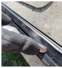
Before installing the hydrophilloc round cord in the profile frame, it should be dry and clean. Press the tip of the tool into the recess provided for the cord in the centre of the profile. Pull along the profile with sufficient pressure.
