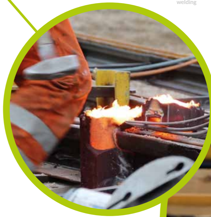
Joint welding of the rails by means of thermite welding
