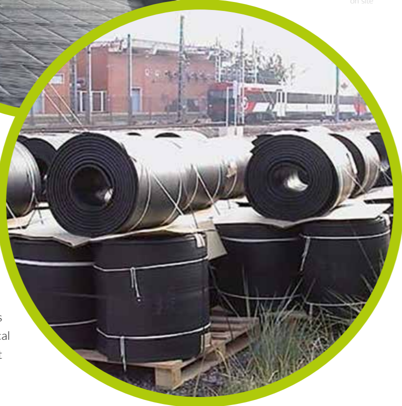
Weather-independent storage of the trackbed mats for fast processing on site
